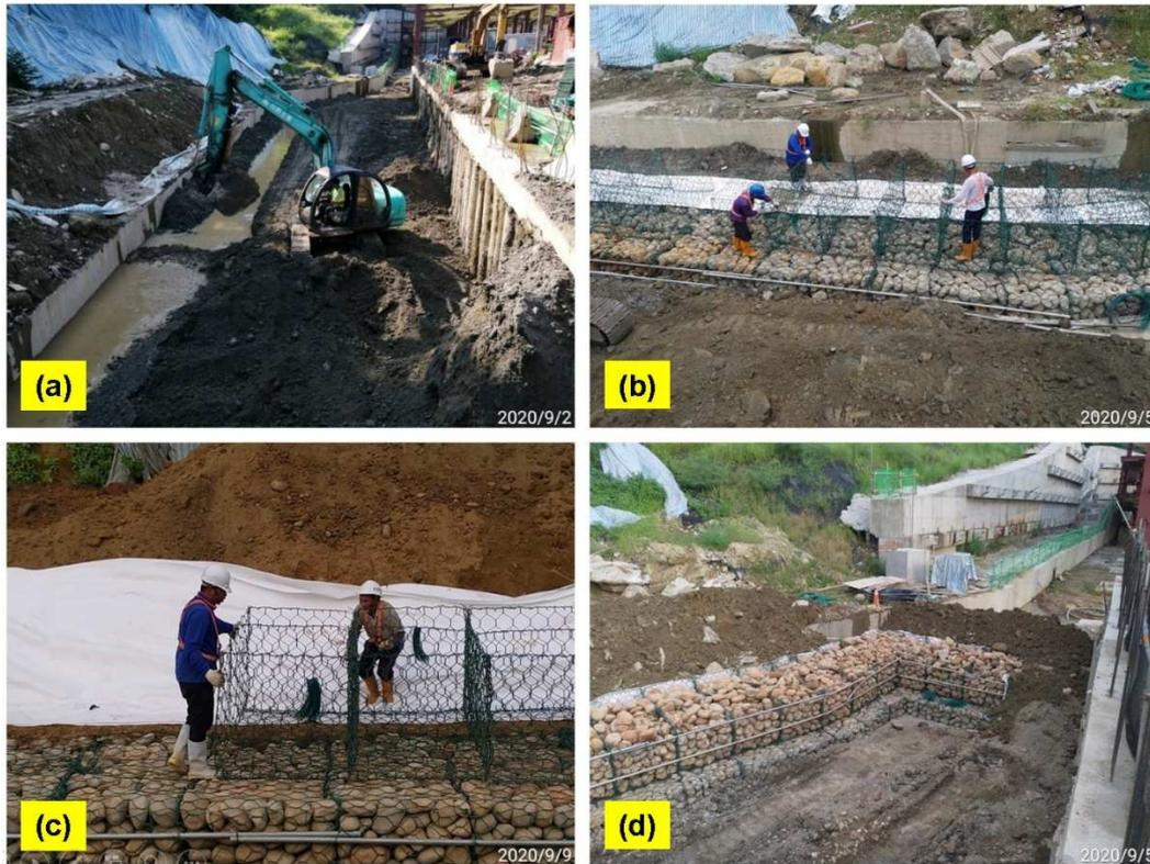
Figure 9 The work processes of the gabion structure: (a) excavation for the pond, (b)&(c) installation for wire mesh boxes, and (d) filling of the gravels
