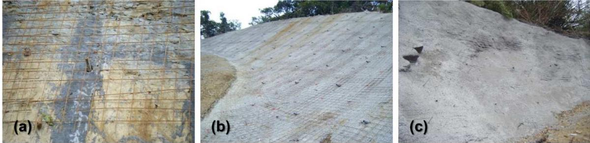
Figure 6 The appearances of the shotcrete structure slopes in different stages: (a) installation of wire meshes and SN anchors, (b) first layer spraying of shotcrete, and (c) finish of final shotcrete slope surface
